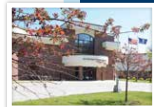
2004 SOAR Center Addition
