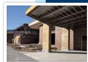
2018-2020 Harrison Campus - Main Building Renovations
